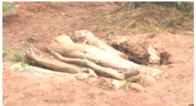
Dan's family latrine made of wood logs with a dug a hole
