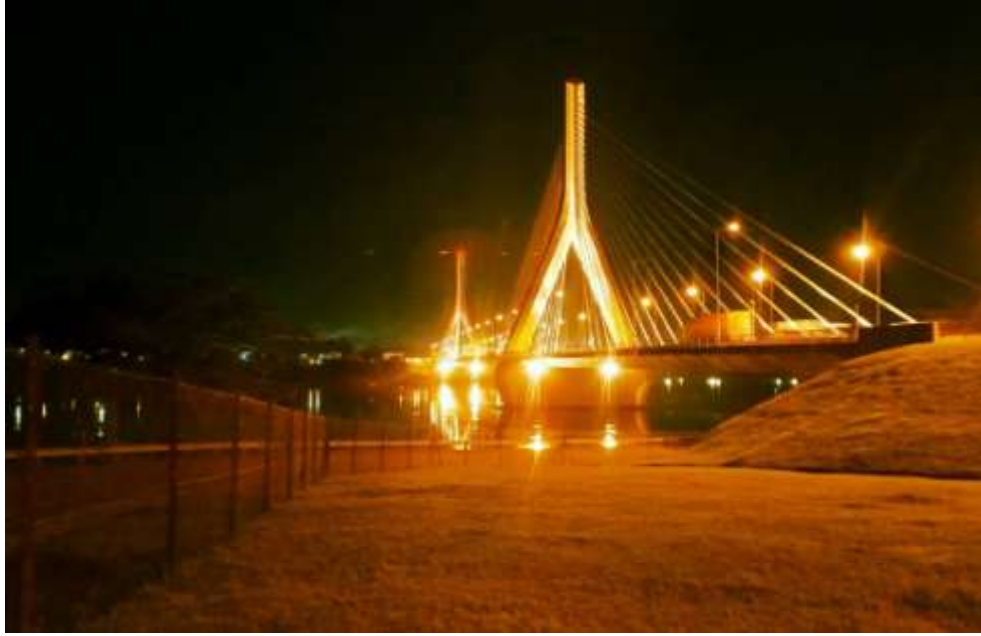
Lighting of the New Jinja Bridge
